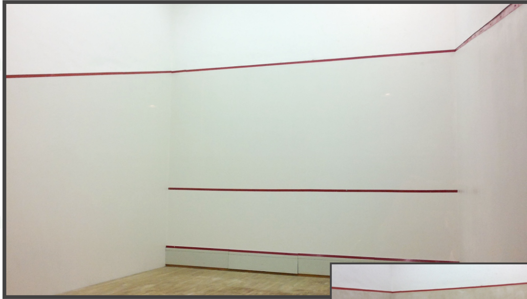
RENOVATED COURT WITH ASB SYSTEM 40
