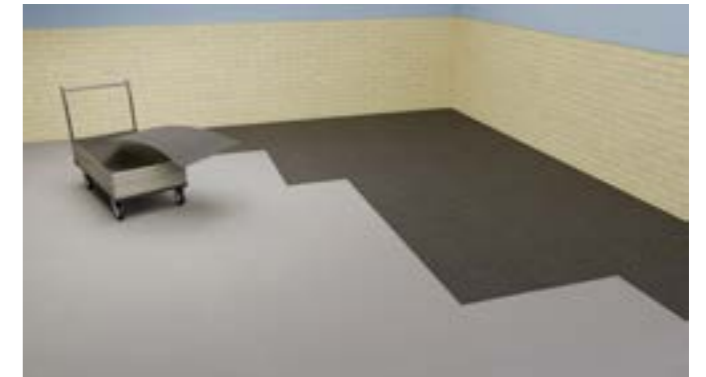
Step 2: Position the Tiles onto the Floor
